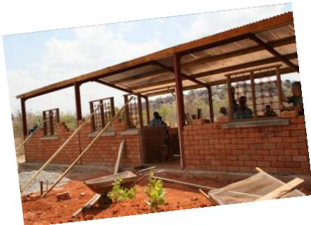
is cast just at the top of the windows. The out side is being pointed at present as are the fixing of the external doors.
