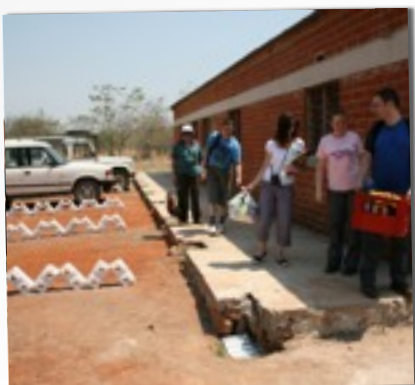
TEAM ARRIVING ON SITE
