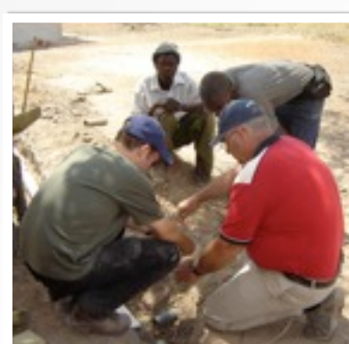
CONNECTING UNDERGROUND CABLES
